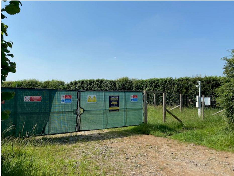
Figure 1: View of entrance to Blenheim Estate's existing solar farm off Banbury Road
